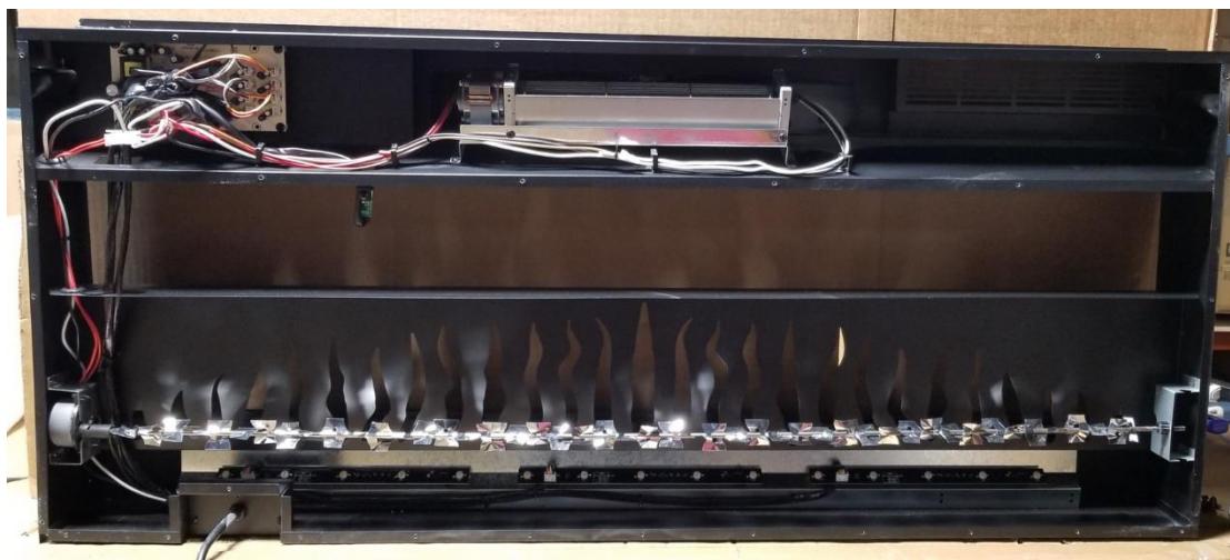
Inside of Fireplace with Back Panel Removed
