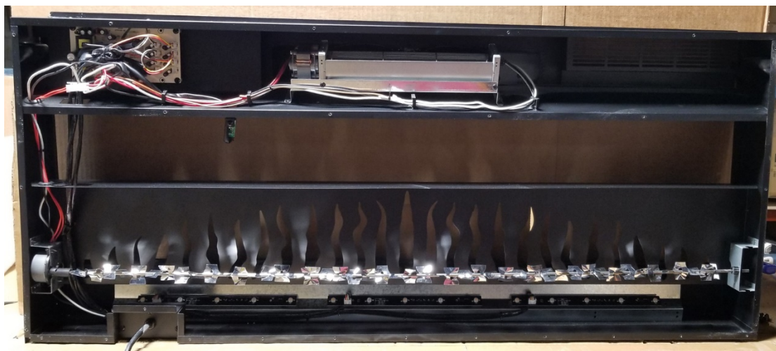
Inside of Fireplace with Back Panel Removed
