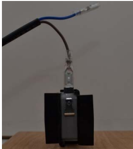
Connect Brown Wire To Top Connection
